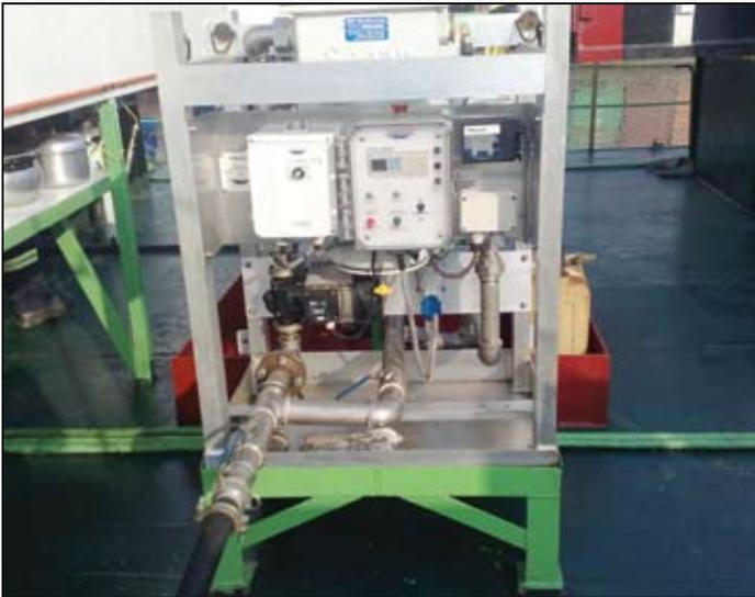
*Fuel Polishing System installed on dredging barge.*
